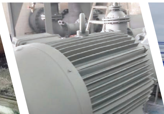
Hydroelectric power plant on the Neretva
