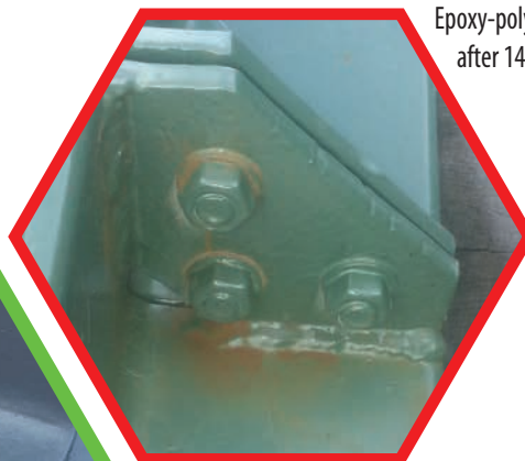
Example of poor surface preparation and subsequent rusting through epoxy primer 3 days after application
