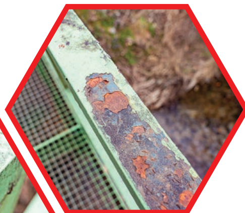
Same bridge, painted with epoxy/polyurethane system, at the same time
